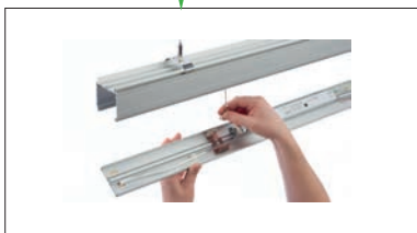
Secure electrical unit to trunking with security cable
