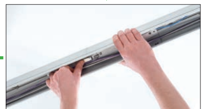
Slide catch over hook to make mechanical fix
